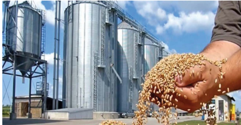
Figure 2. Array of large vertical steel silos for grain storage.
